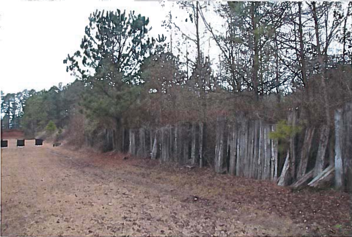
Photo 7: Existing Rifle Range - North Berm Near Firing Line
